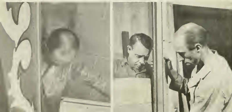
BELOW: STAGE HANDS MATCH "TONGUE AND GROOVE" OF SCENERY UNITS IN SYSTEM DEvised BY NBC FOR THE RAPID ERECTION OF TELEVISION STAGE SETTINGS.
